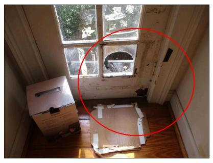
(4) The exterior door leading to the dining room (at rear of home) revealed multiple signs of wood rot and moisture intrusion. Further damage will occur if not repaired. Recommend a licensed contractor make all needed repairs.
