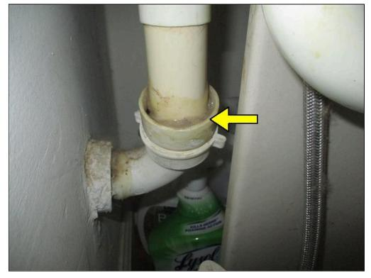
(6) Plumbing waste line drains slowly at the upstairs bathroom sink. A cause of a slow drain can range
