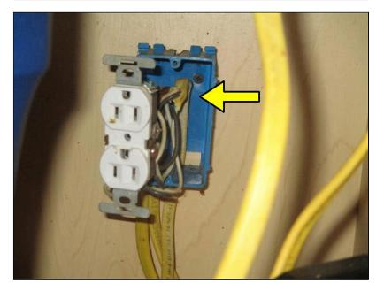
(7) There are exposed wires under the gas cooktop in kitchen. Recommend an electrician repair.
