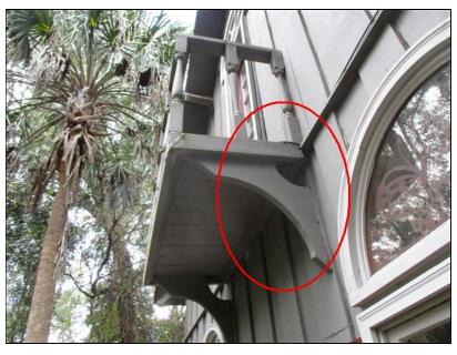
(3) The porch overhang at the left rear of home appeared to be in overall poor condition. There were signs of wood rot and failure in areas. Recommend a qualified contractor inspect further and make all needed repairs or replacements.
