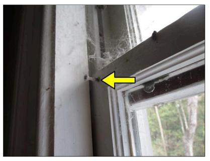
(4) Most if not all the windows were stuck or painted shut. I was unable to open any of the windows during the inspection. Recommend repair.
