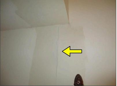
(2) Sheetrock walls have normal cosmetic defects at most if not all rooms. Nail pops and minor cracking is to be expected in a home while it settles. If condition worsens, then a qualified contractor should inspect further and repair as needed.
