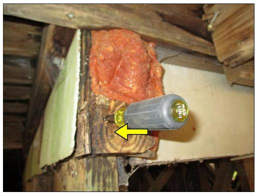
(2) The balcony at the upstairs bedroom is weak and failing. The pickets were missing in areas or were too wide, and the overall structure was weak and appeared to be pulling away from the home. Further damage, including failure, could occur if not repaired. Recommend a qualified professional make needed repairs and replacements.
